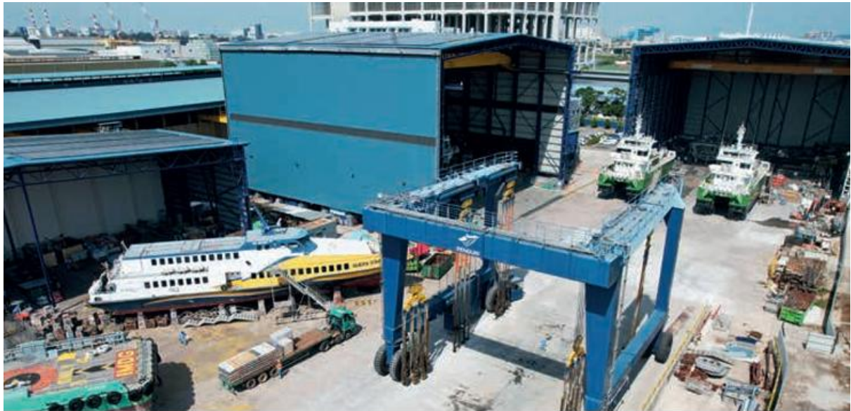
Penguin Shipyard International in Singapore: A hub of bespoke aluminium shipbuilding, ship repair, as well as special conversions and upgrades.
