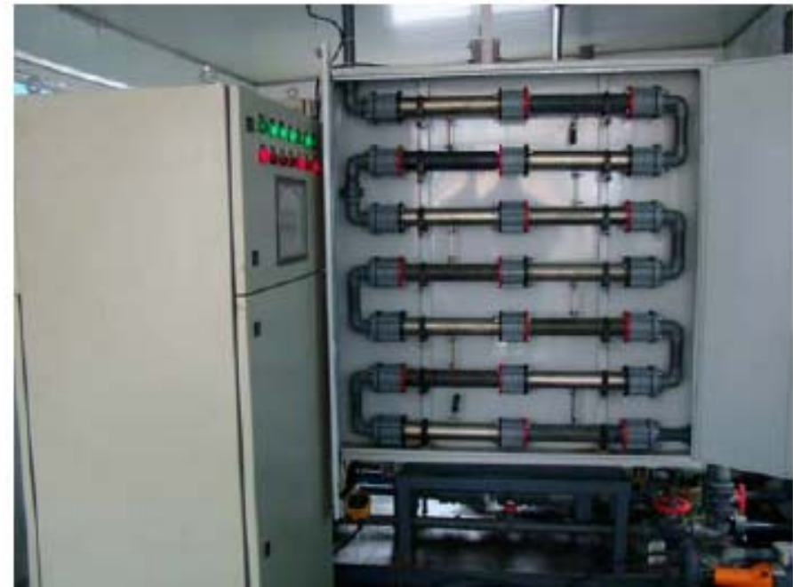
Sunrui electrolytic unit
