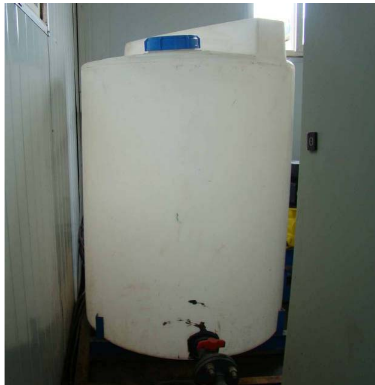
The neutralizer tank
