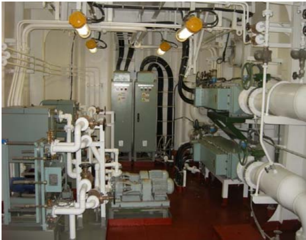
Chemical Tanker - On-Deck Installation
