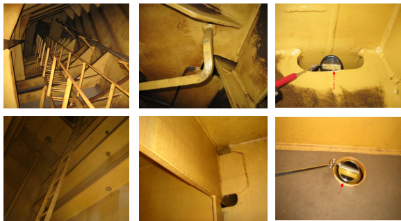
Fig.20 Condition of Ballast Tank Specified with S-I-P
