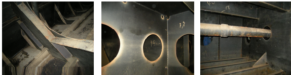
Fig.19 Condition of Ballast Tank Specified with non S-I-P
