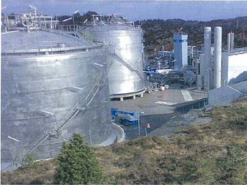
Figure 24: Atmospheric LNG tanks at the Kollsnes LNG plant, Norway. The tanks are 4000 and 2000m 3 . Photo: E.Jarlsby
