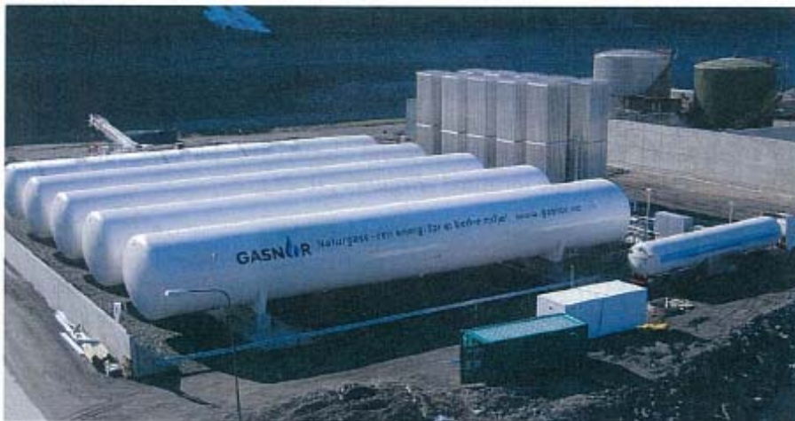
Figure 22: LNG terminal at Mosjøen aluminium plant, Norway. 5 x 683 m 3 pressurised tanks. Photo from Gasnor.
