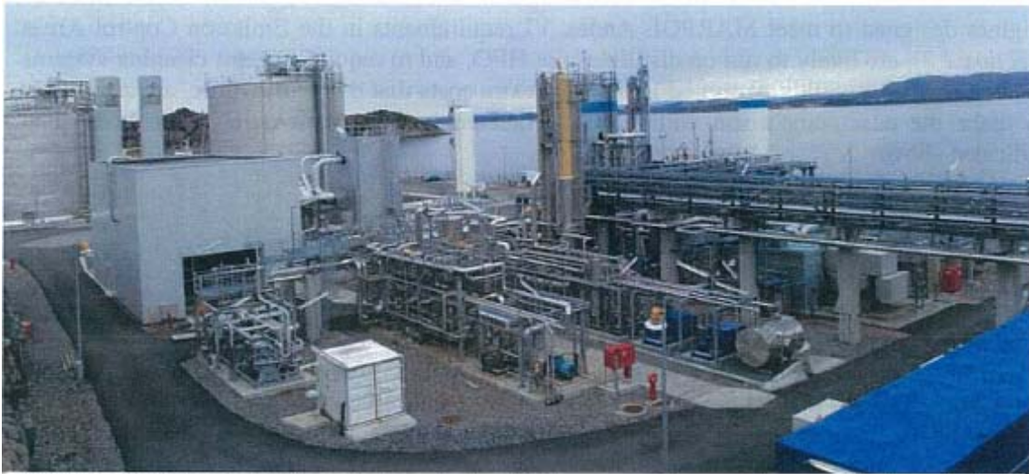
Figure 8: Small scale LNG production plants at Kollsnes, near Bergen, Norway. The two plants at this location have a combined annual capacity of 120,000 tonnes of LNG. Photo from Gasnor.
