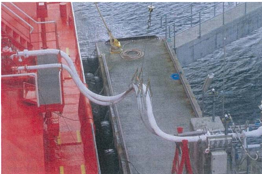
Figure 20: Flexible hoses for loading and discharging the 1100 m 3 LNG carrier "Pioneer Knutsen". The two hoses are for LNG transfer and vapour return. Photo from Gasnor.
