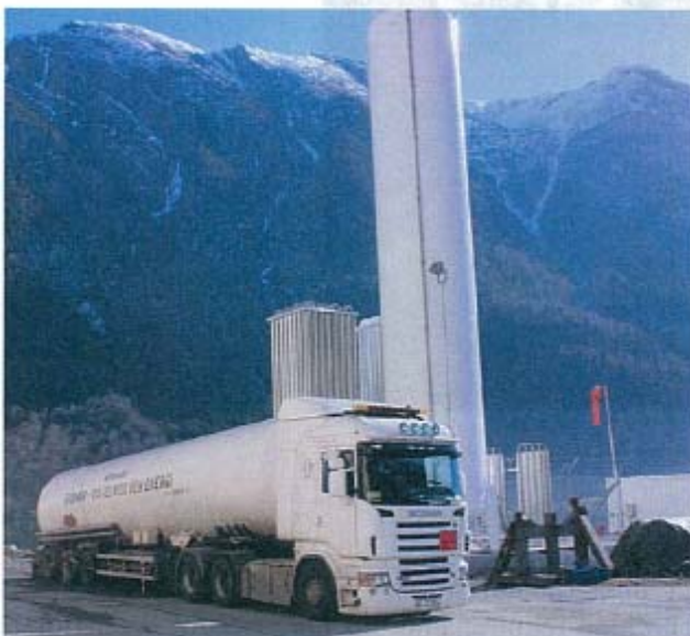
Figure 23: Vertical LNG tank at a small terminal for truck operations. Photo from Gasnor.
