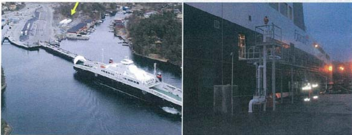
Figure 19: LNG bunkering arrangement from permanent tanks for the coastal ferries at Halhjem, Norway. Photos: Gasnor
