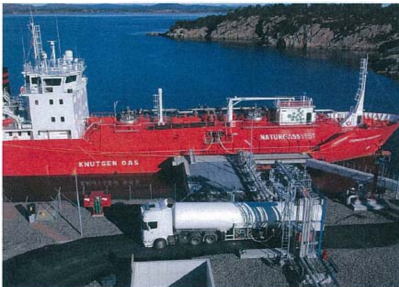
Figure 21: Loading operations for both ship and tanker truck at the Kollsnes LNG plant, Norway. Photo from Gasnor.
